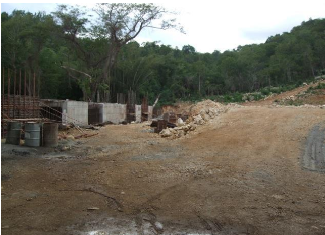
Figure A2 – 7. North-South Highway 2000 Construction
