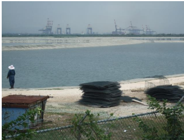
Figure A2 – 14. Soapberry Wastewater Treatment Plant (2)
