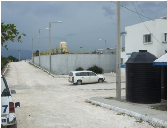
Figure A2 – 37. Soapberry Wastewater Treatment Plant
