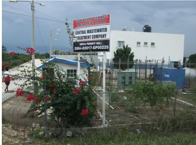
Figure A2 – 13. Soapberry Wastewater Treatment Plant (1)
